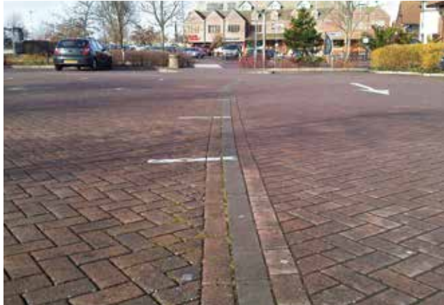
Figure 8.4 Lined permeable pavement constructed over a former landfill site, Portsmouth (courtesy EPG Limited)
