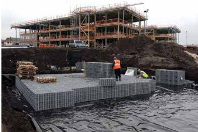
Figure 21.1 Geocellular storage system under construction (courtesy Polypipe Limited)
