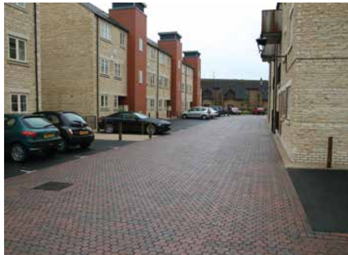
Figure 8.2 Unlined permeable pavement on a contaminated site, Stamford, Lincolnshire (courtesy EPG Limited)
