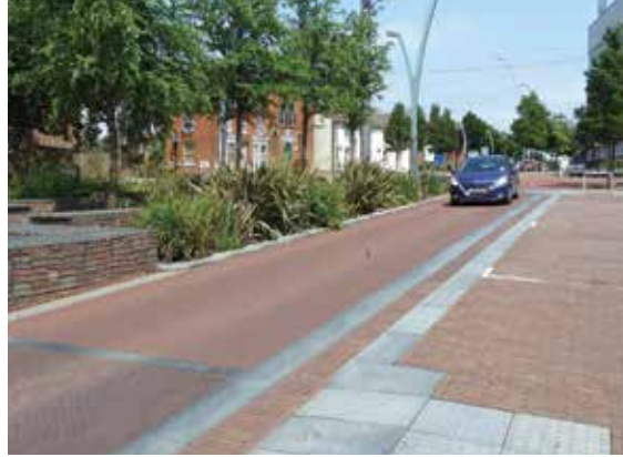
Figure 9.9 Bioretention system, inner ring road around Ashford town centre (courtesy Kent County Council)
