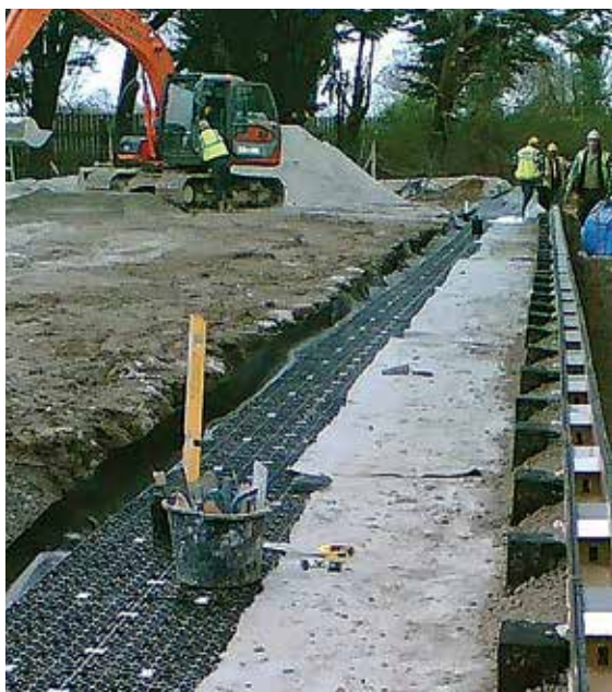
Figure 14.2 Treatment channel installations showing discrete 1 m sections (courtesy Permavoid Limited)
