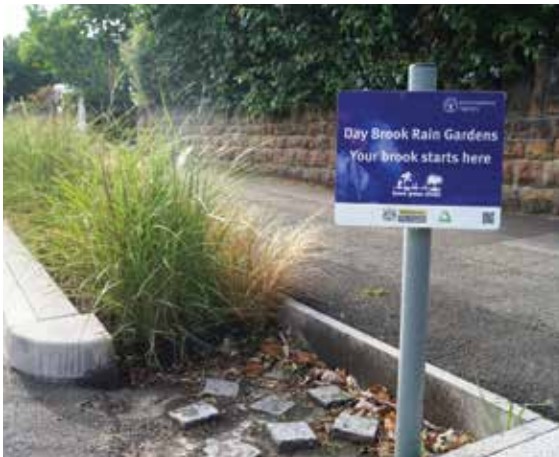
Figure 18.11 Example of a bioretention system with a simple sediment forebay, Nottingham (courtesy Environment Agency)
