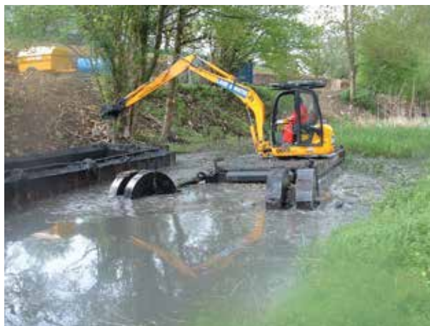
Figure 32.3 Floating excavator working in small pond (courtesy Land & Water)
