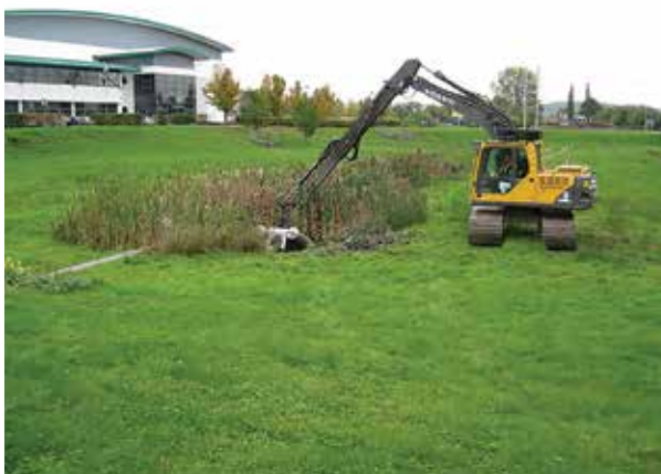
Figure 32.2 De-silting (courtesy Bedford Group of Drainage Boards)
