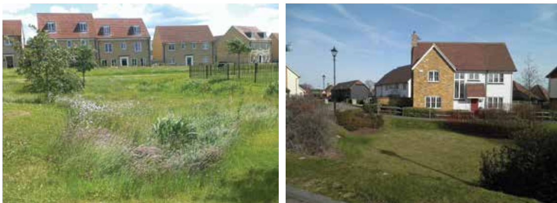
Figure 22.6 Examples of detention basins with easy access for maintenance (courtesy Peterborough City Council and Kent County Council)
