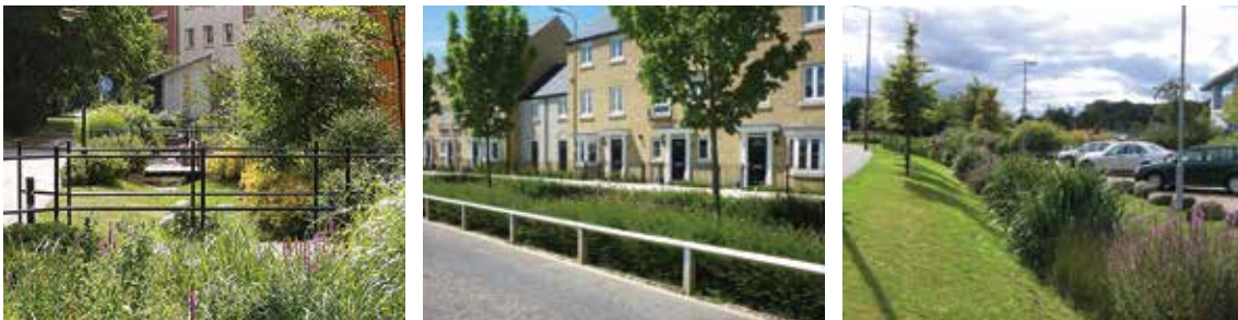
Figure 10.6 Swales and linear wetlands (courtesy Essex County Council, Leicester City Council)
