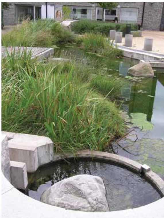
Figure 23.7 Pond with baffles and islands, Augustenborg, Sweden
