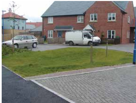
Figure 13.7 Small infiltration basin, Cambourne (courtesy Illman Young)
