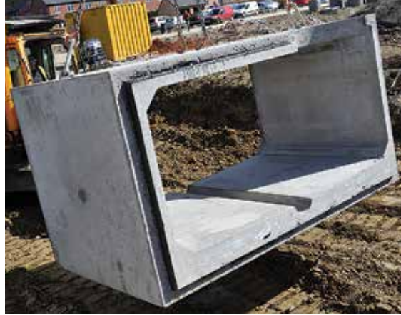
Figure 21.13 Precast concrete box culvert being installed as part of a SuDS scheme (courtesy British Precast)
