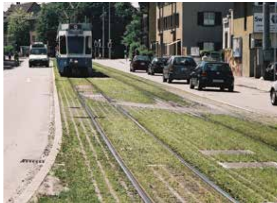
Figure 9.2 Concrete grid grass reinforcement along tramlines, Switzerland (courtesy EPG Limited)
