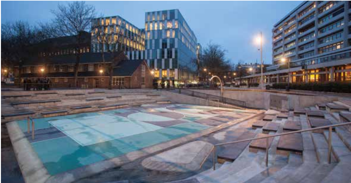
Figure 22.5 Example of urban hard surfaced off-line detention basin with geometric design to enhance amenity use, Rotterdam, the Netherlands (courtesy pallesh+azarfane)
