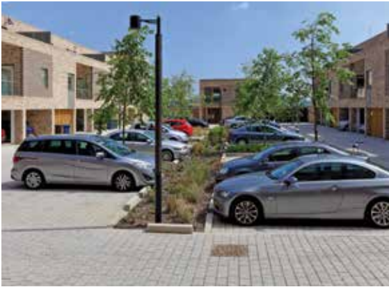
Figure 9.1 Concrete block permeable paving used for a residential road, Cambridge (courtesy Cambridge City Council)
