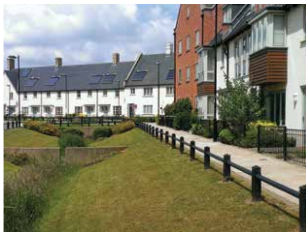
Figure 17.8 Dry swale with overlying flow control, Upton, Northamptonshire (courtesy Peterborough City Council)
