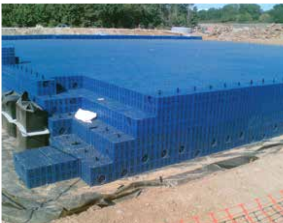
Figure 21.2 Structural frame being constructed (courtesy EPG Limited)
