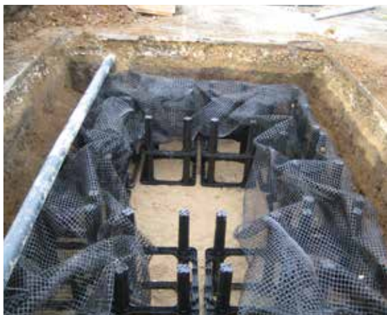
Figure 19.8 Placement of modular structures in a tree pit (courtesy Consulting with Trees)
