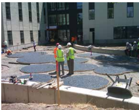
Figure 20.6 Construction of pavement using resin bound post consumer recycled glass aggregate (courtesy Filterpave Limited)
