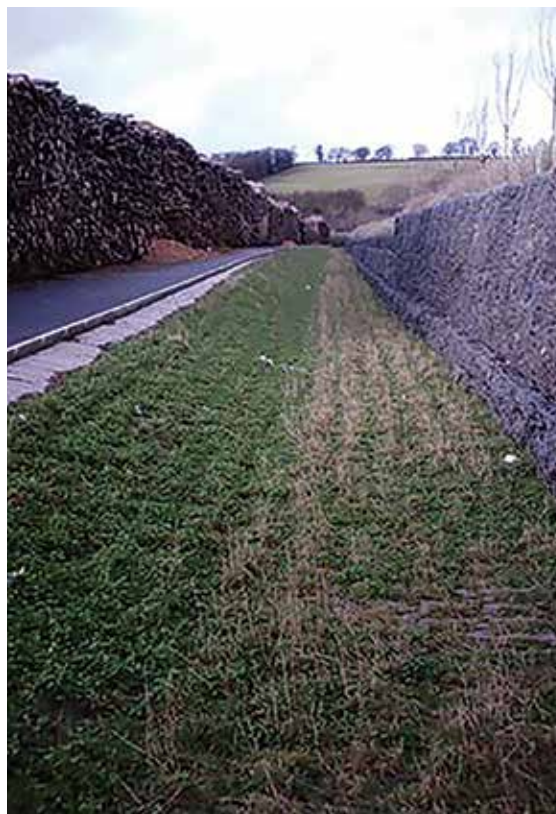
Figure 17.6 Swale with vertical side (courtesy EPG Limited)
