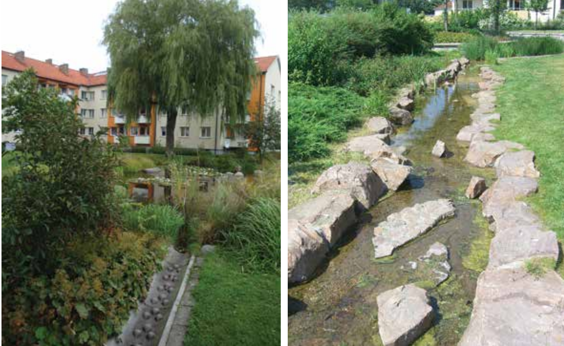
Figure 23.12 Energy dissipating inlet channels for ponds, Augustenborg, Sweden (courtesy Graham Fairhurst and Illman Young)
