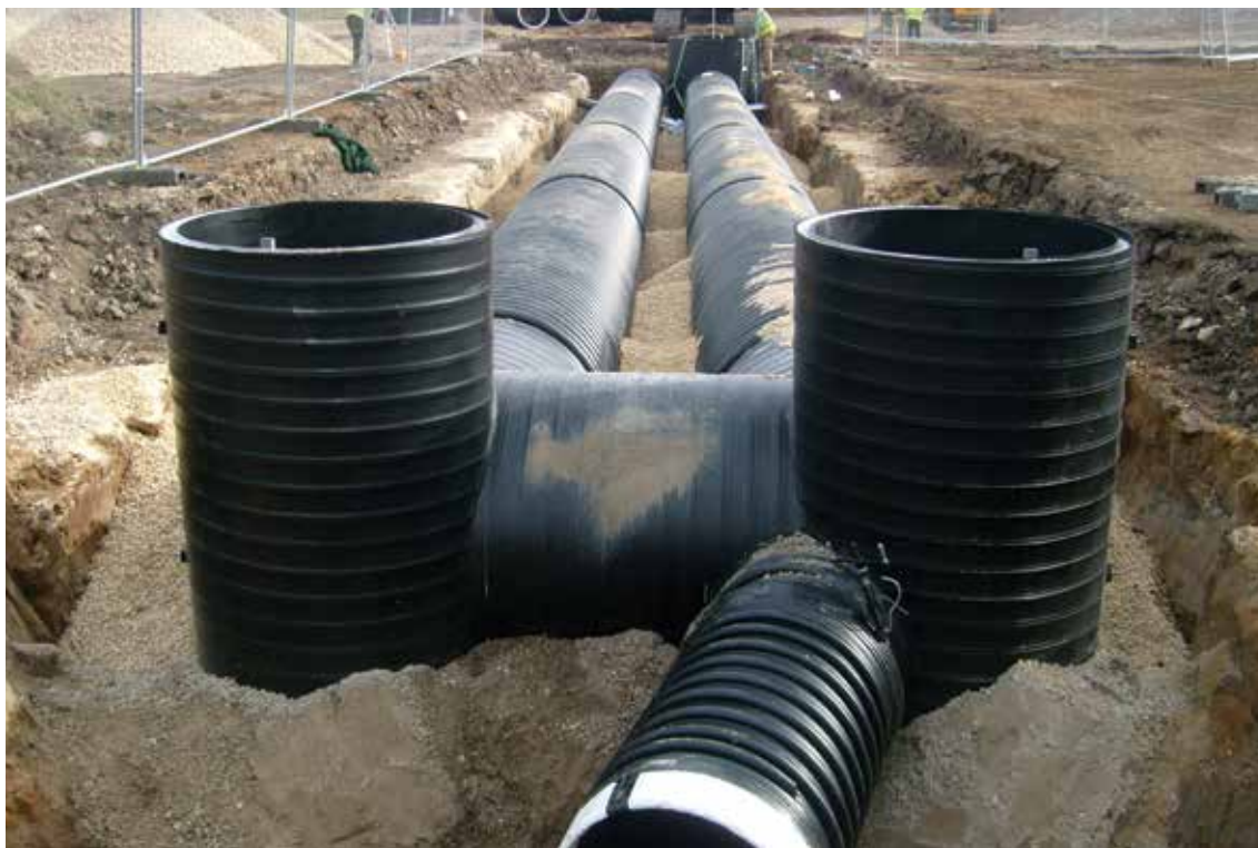
Figure 21.11 Installation of oversized plastic pipe attenuation tanks (courtesy Polypipe Limited)
