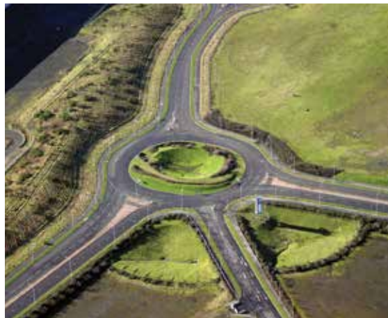
Figure 22.4 Detention basin in a roundabout, DEX, Dunfermline (courtesy Abertay University)
