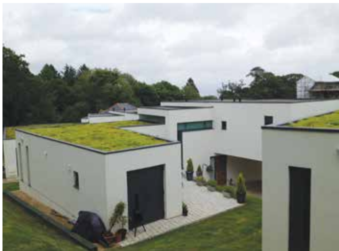
Figure 12.5 Domestic green roofing, Swansea (courtesy Sky Garden)
